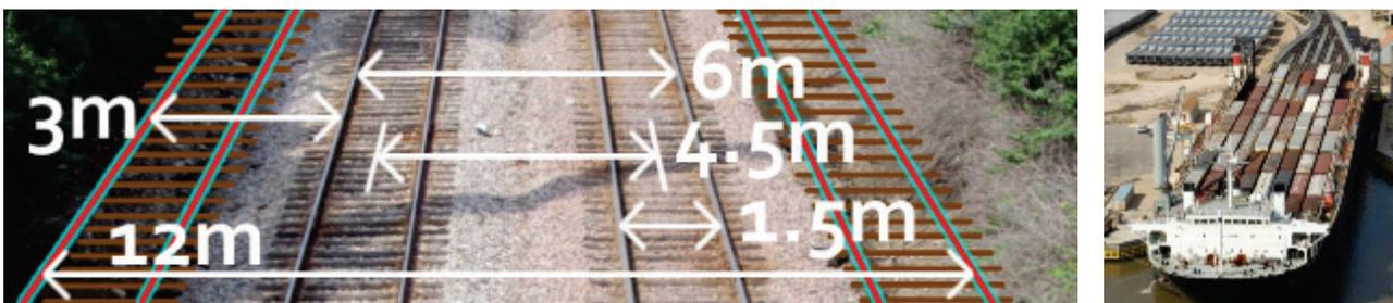
Rolling between ship and shore is aided by ballast tanks on ship, which align height of ship to that of shore, an example of which is pictured above-right.
