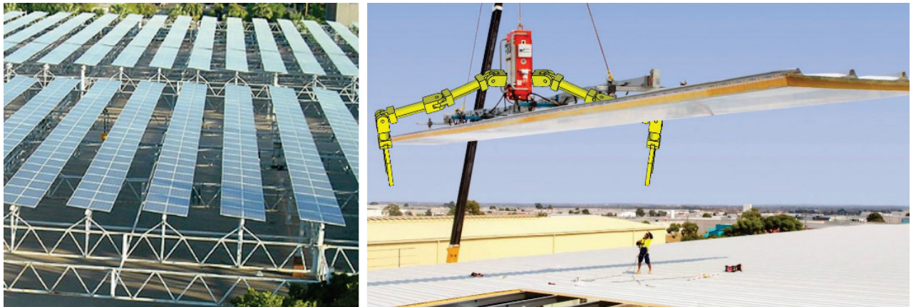
Figure 15.3. Standardized sub-assemblies with automated assembly (concept illustration by Weinreb).
