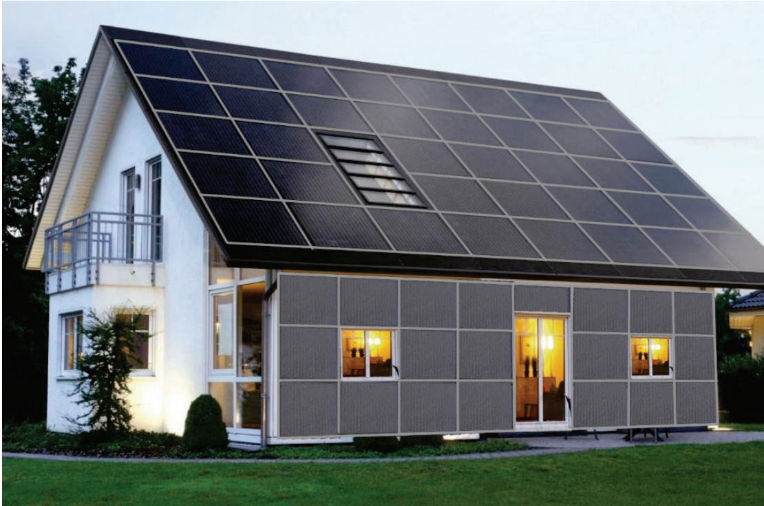
Figure 14.1: Illustration of custom PV solar skin that mounts directly onto plywood and wraps features such as windows and doors (concept illustration by Weinreb).
