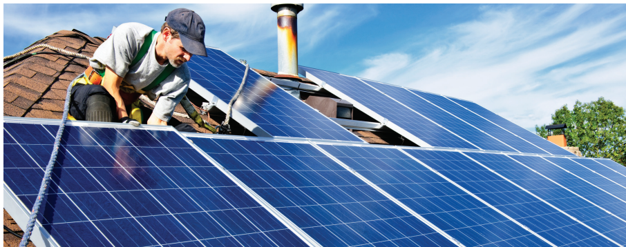
Figure 21.4: Residential solar panel installation.
